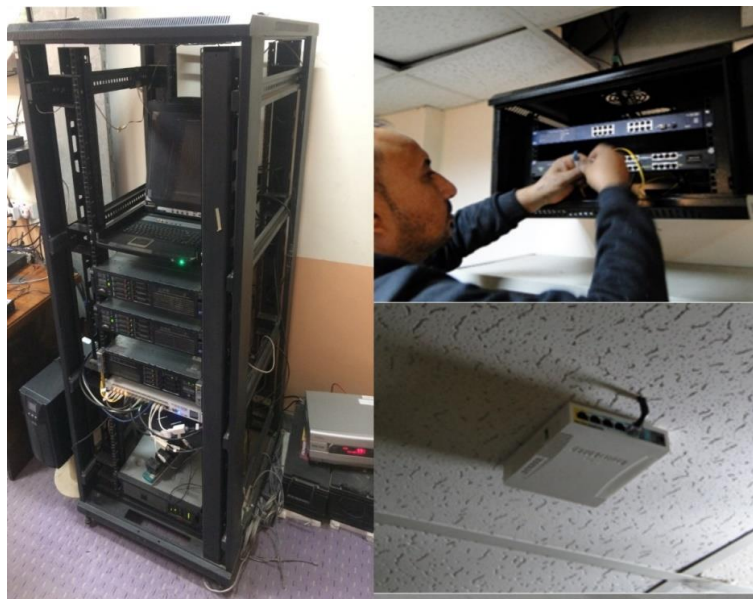
Fig. 2. Fiber optic and Wi-Fi installation.
