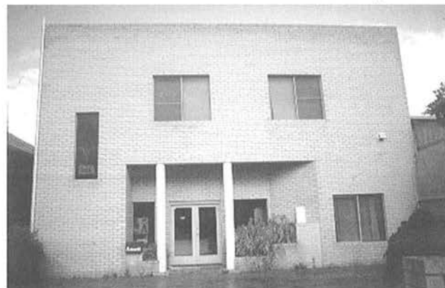
Office warehouse, East Perth.
