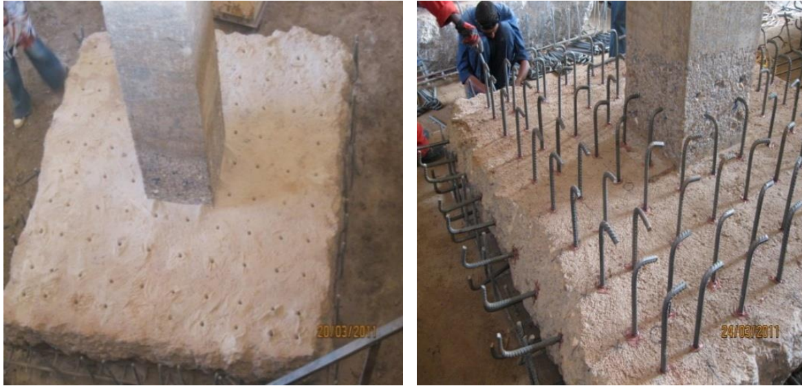
Fig 5. Drilled holes and inserted dowels bars.
