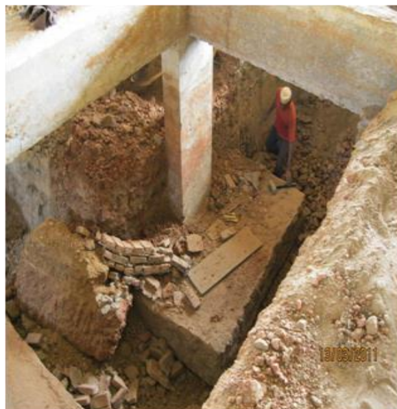
Fig 4. Excavation around the footing.
