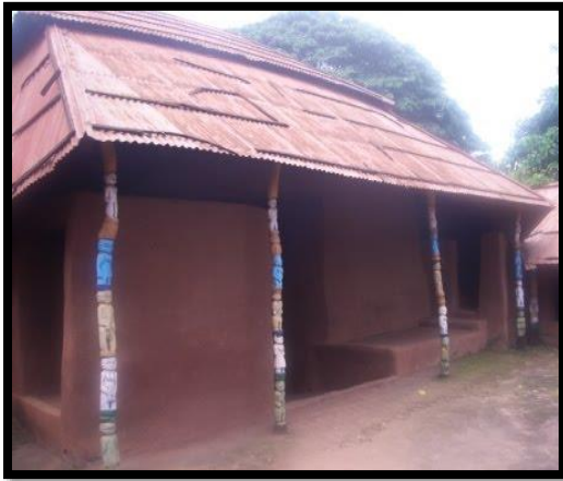
Figure 3. Entrance façade of a traditional building.
