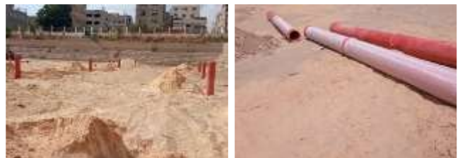
Figure 4: Borehole drilling and UPVC pipes installation at Waqf basin
