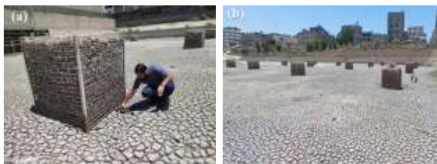
Figure 7: Graveled borehole gabion at Waqf basin: (a), (b)
