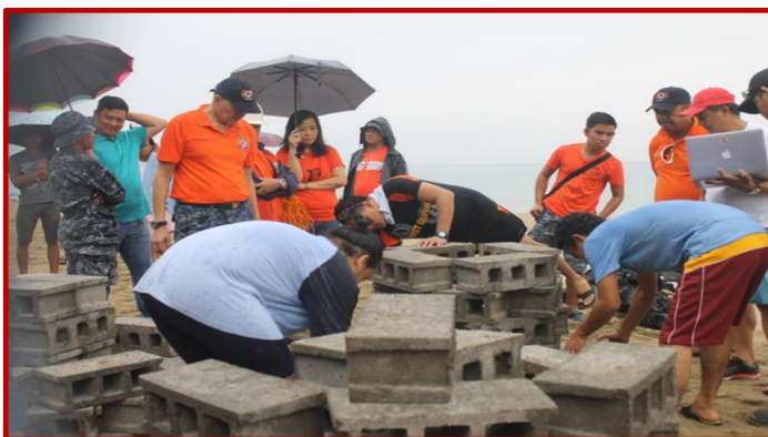
Plate No. 2 Onsite preparation
