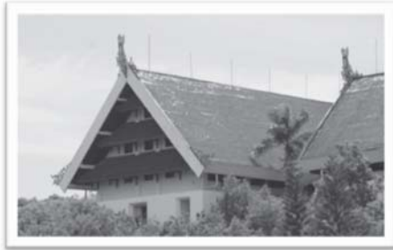
Picture 1. Office of the Governor of South Sulawesi Province is characterized by applying a roof Anjong Bugis (Photo: Pangerann PY, 2012)
