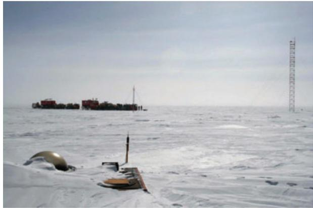
The expedition stopped at Plateau Station, last occupied by US scientists in 1969. The tall meteorological tower and some smaller towers are still standing. The clear dome of the aurora tower and the top of a smokestack of the old main station are visible just above snow level. The Norwegian–US team entered through a hatch and found the buried station to be a time capsule of the late 1960s. (Photo by Stein Tronstad; courtesy of Norwegian Polar Institute Photo Library.)
