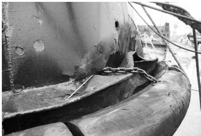
Rys. 2. Uszkodzenie dziobu (forepik i nadburcie) Fig. 2. Damage to the bow (forepeak and bulwarks)
