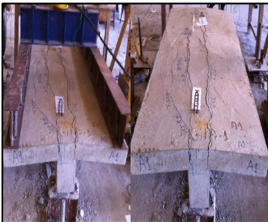
Figure 16. Mode of failure of specimen GIM-4.
